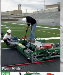
Fully automatic paver for elastic layers, elastic subbases, athletic tracks and multipurpose sports surfaces.
