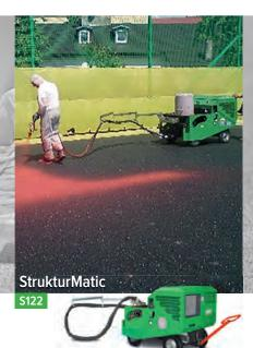
Spraying machine for structured spray coatings and primer.
